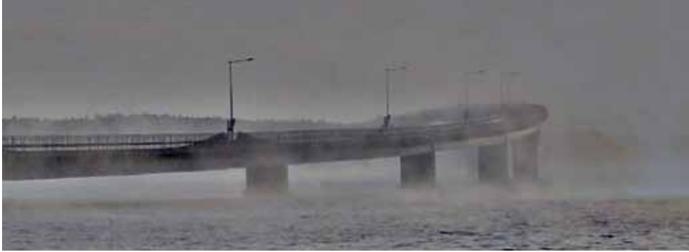
The bridge to and from Torsö.
