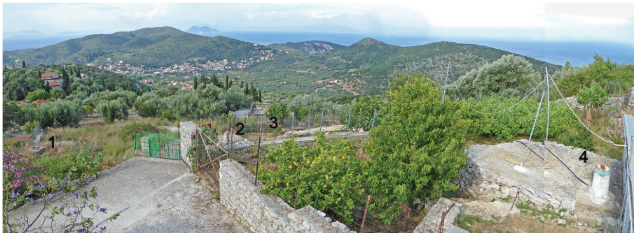
Photo 7: Ithaca landscape with four rainwater tanks
