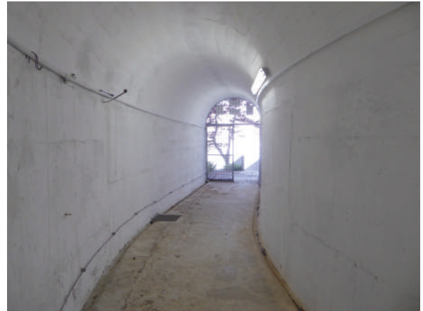
Photo 4: Tunnel leading to the spring deep into the mountain
