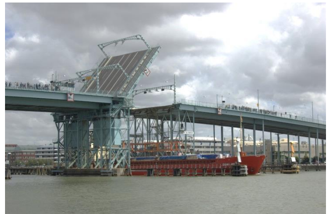
The Götaälv Bridge in Gothenburg.
