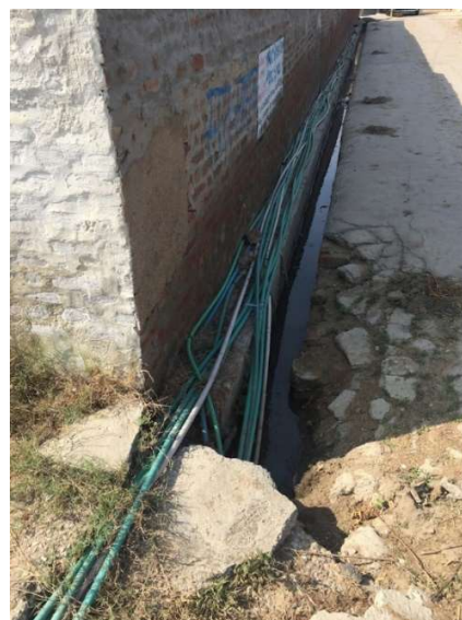
Figure 9: Section of the informal semi-covered network of PVC pipes developed by the private water seller.
