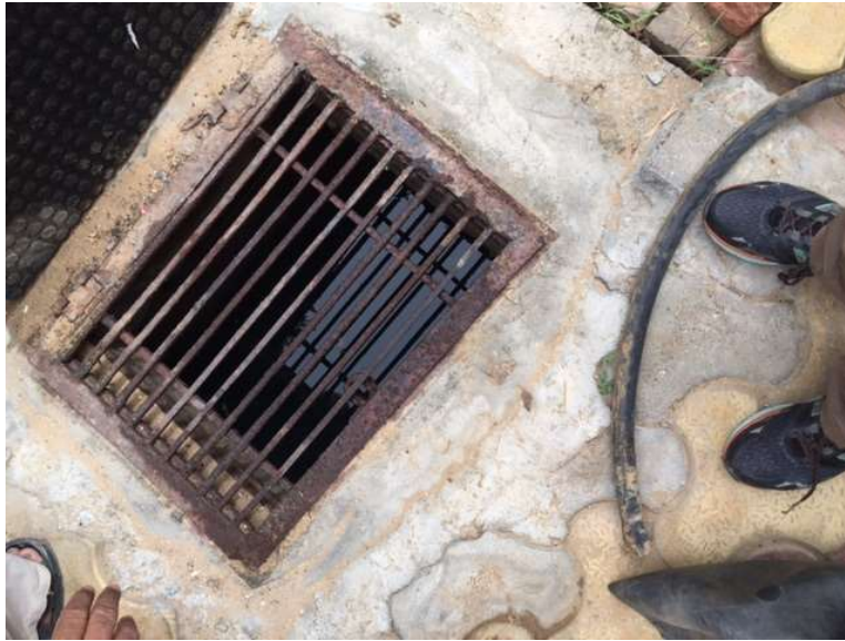
Figure 2: Underground storage tank in a private bungalow in the upstream part of the village
