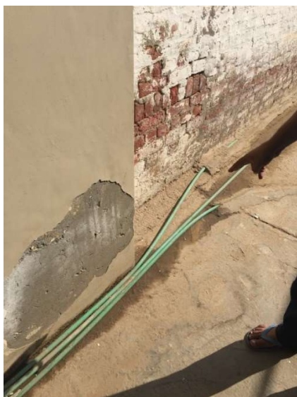
Figure 9: Section of the informal semi-covered network of PVC pipes developed by the private water seller.
