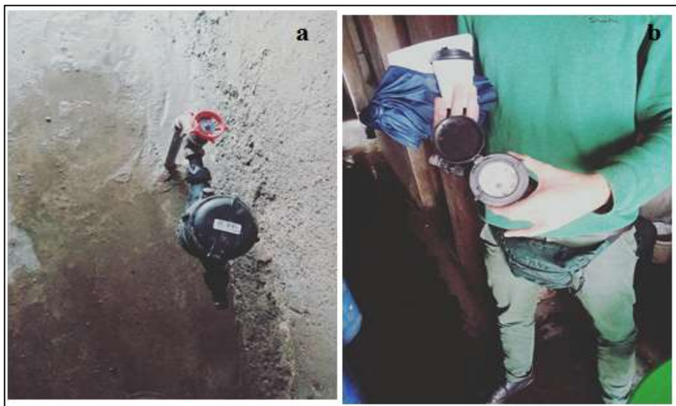
Figure 3: Examples of Jisomee Mita in an assembled state (a) and removable state (b)
