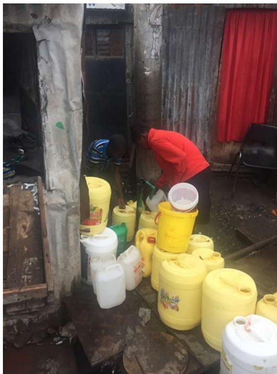
Figure 5: Illegal water connection in the Mathare settlement.
