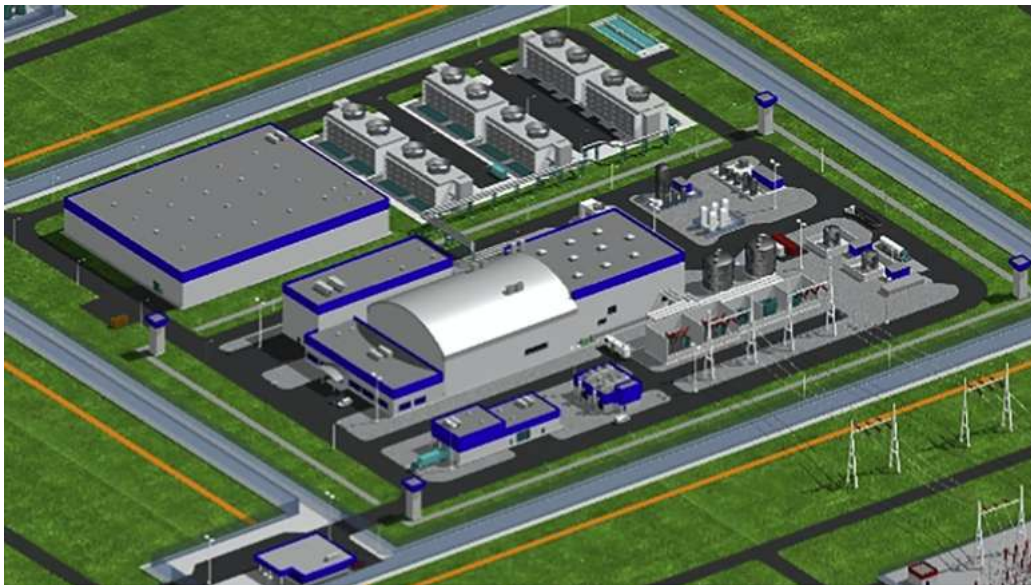
Figure 1.10: Westinghouse LFR plant layout [33].
