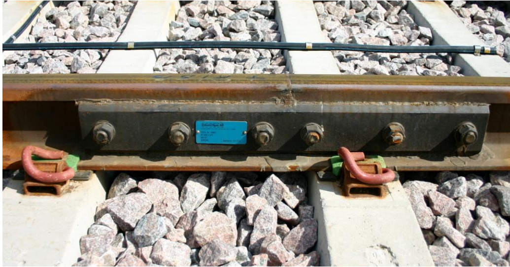
6-hole prefabricated insulated joint
