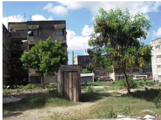
2 Group of Apartment Blocks with Tenants' illegal Pit-latrine Block in forecourt
