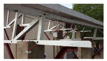
Figure 8 : Fixation to the pillars
