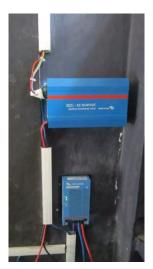
Figure 10 : Inverter and charge controller
