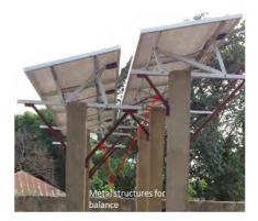
Figure 9 : Structure reinforcement
