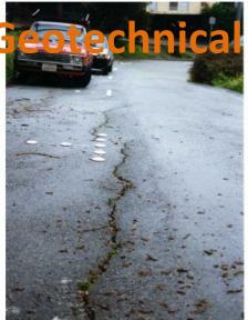
En echelon cracks in asphalt pavement caused by slip on the Hayward fault.
