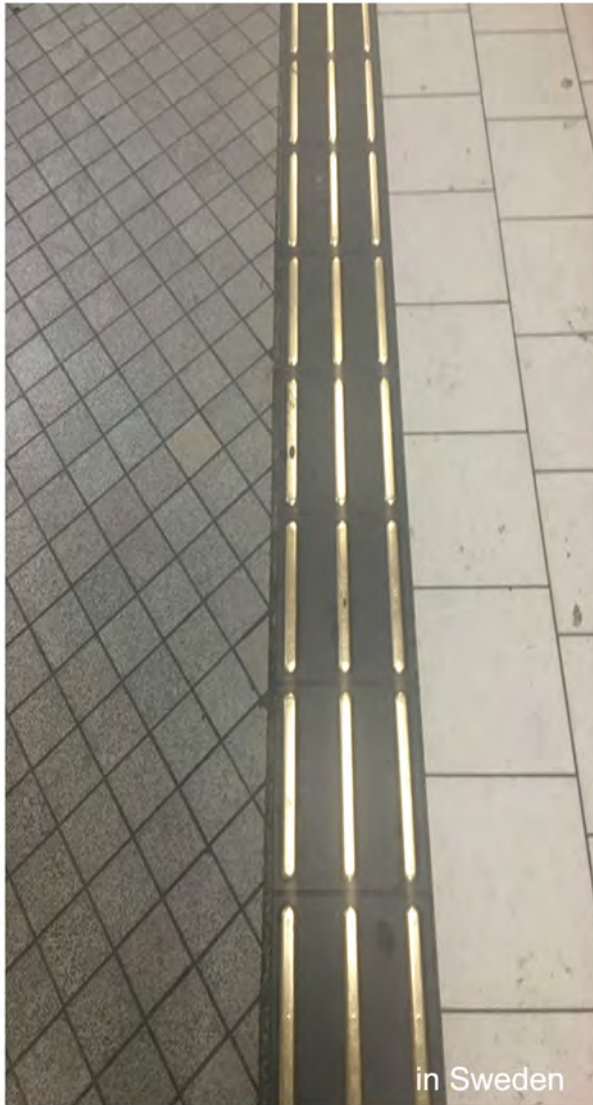
( the photo taken by myself at metro station of Stockholm)
