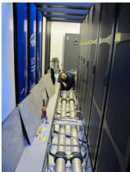
Left: Beskow is water-cooled and requires a substantial amount of water. Here new pipes are being installed for Beskow under the old Cray, Lindgren.
