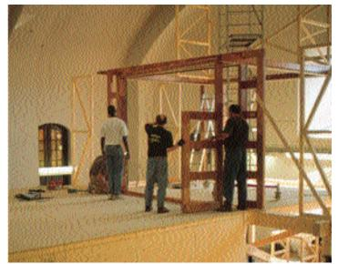
**Above:** Members of the TAN construction crew attach the door to the frame of the Cube. Because the door is one of the image surfaces and must also open and close, it is hinged on the outside using wooden hinges.
