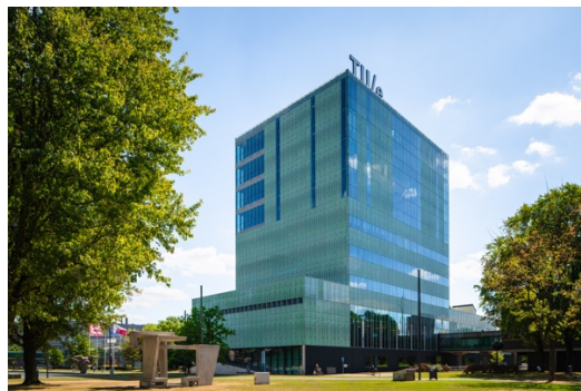
Department of the built environment
