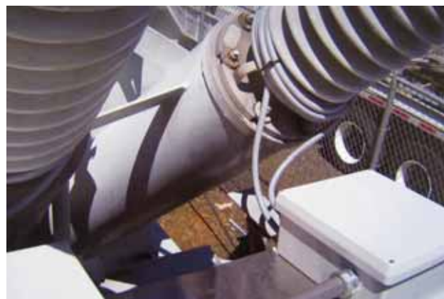
Figure 6.23: Alstom COSI-NXCT F3 flexible optical current transformer in a portable substation application
