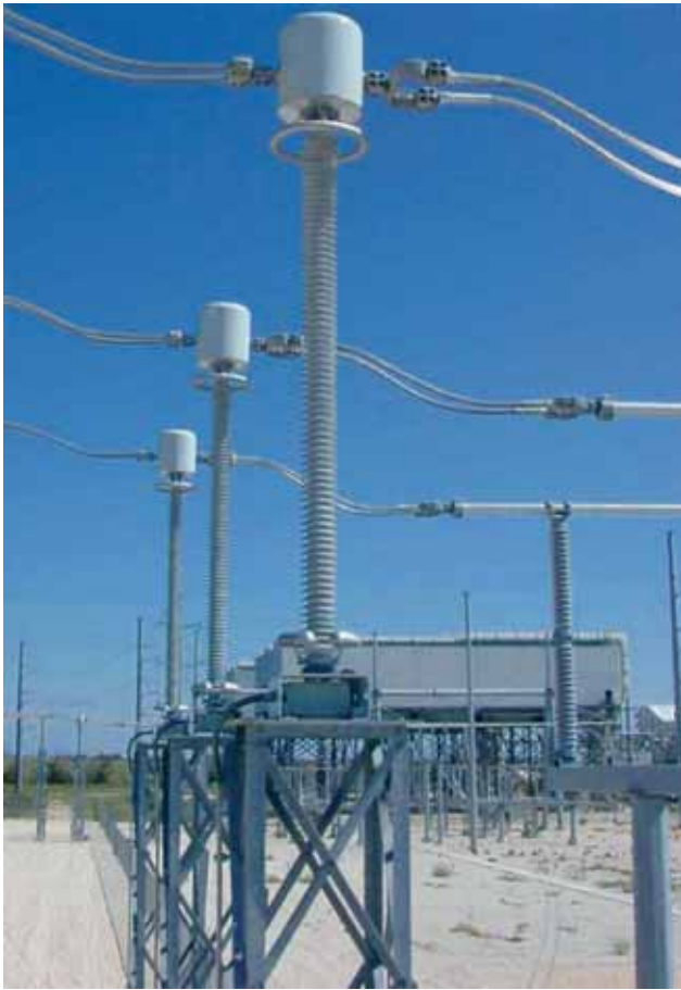
Figure 6.25: Installation of a CT with an optical sensor
