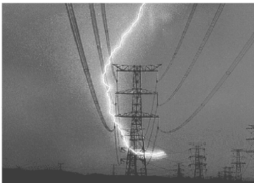
Left: Photograph of an UHV transmission line struck by lightning. Right: Example of a real power transmission line in a complex topography
