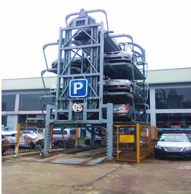
Figure 2.2: Rotary type automated car park in downtown Brooklyn. Source: Park-matic
