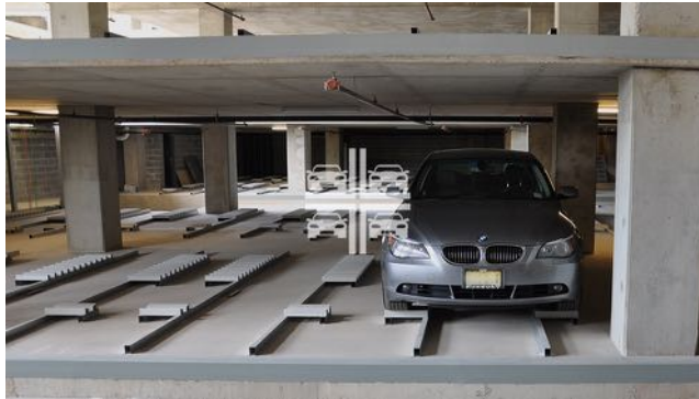
Figure 2.8: Non-pallet solution with carts lifting the wheels of the car by coming in between the combs. Source: Park Plus
