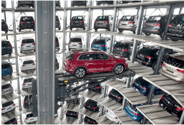
Figure 2.1: Volkswagen's elevator typed automated car collection system in Autostadt, Germany. Source: autostadt.de
