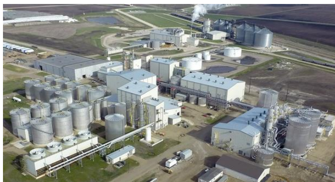
Figure 1. Poet-DSM Project Liberty is a cellulosic ethanol plant using engineered yeast, together with many other technological advances, to produce renewable biofuel from corncobs, leaves, husk and stalks. Image: dsm.com
