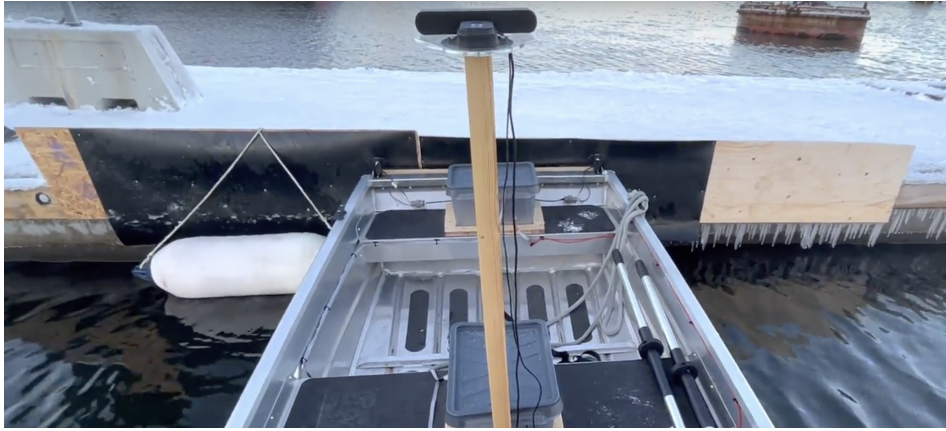
Figure 5.3. The constructed dock covered in a rubber sheet.
