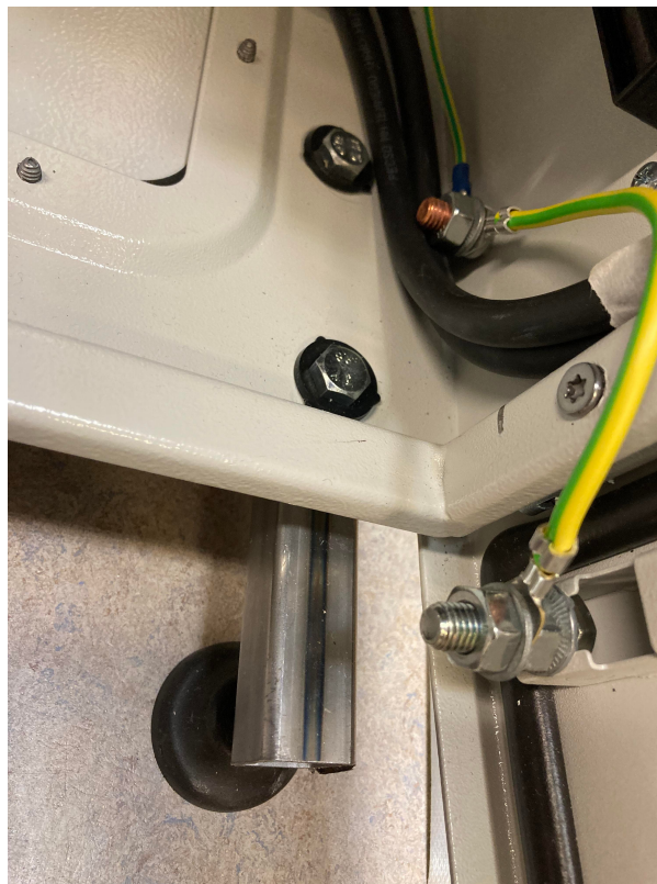
Figure 4.2: Mounting of RSU feet
