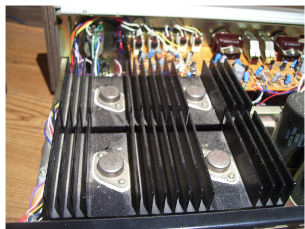
Large heatsinks to cool power transistors in a TRM-800 audio amplifier
