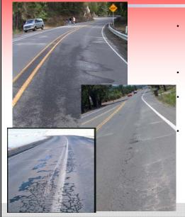
Description: Water bleeding (left two photos) occurs when water seeps out of joints or cracks or through an excessively porous HMA layer. Pumping (right-most photo) occurs when water and fine material is ejected from underlying layers through cracks in the HMA layer under moving loads.
