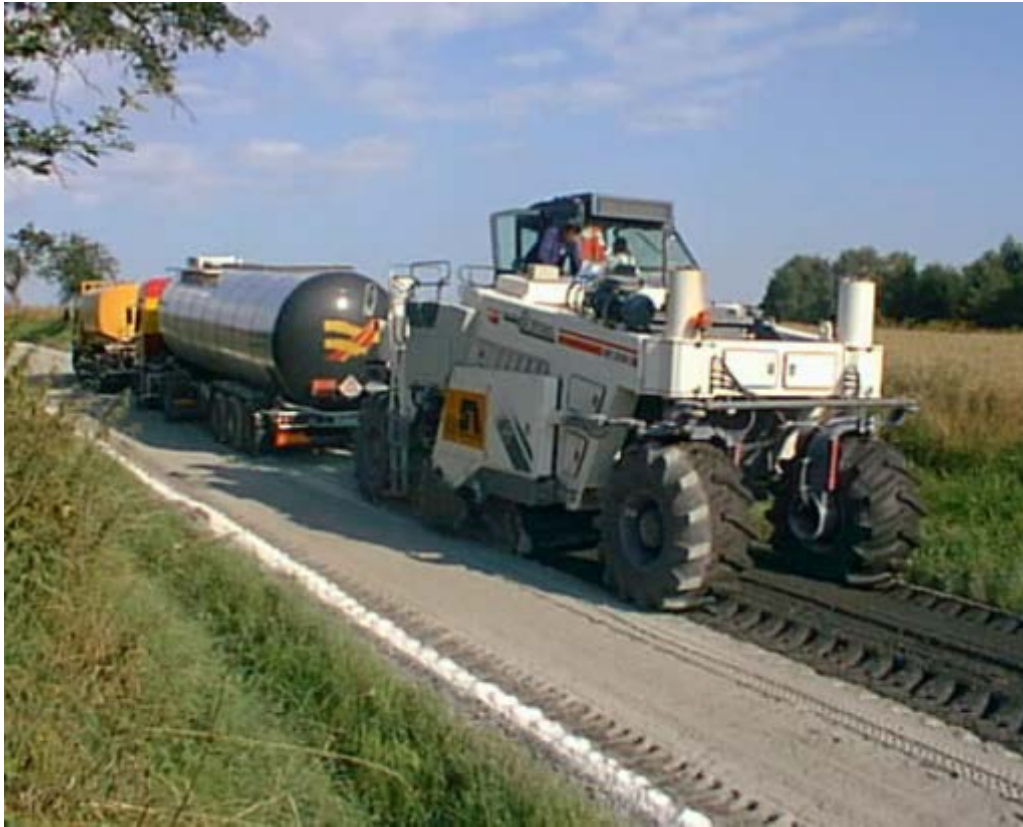
FDR WITH FOAMED ASPHALT
