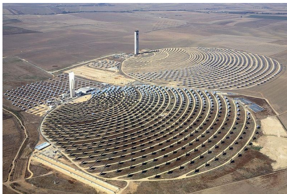
The solar park with the two towers receiving the sunlight from the large parabolic mirrors. (by courtesy of Solar Millenium)
