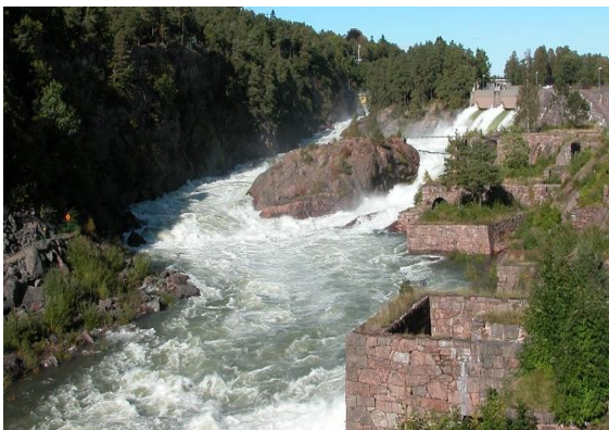
Power plant at the Trollhättan waterfalls.
