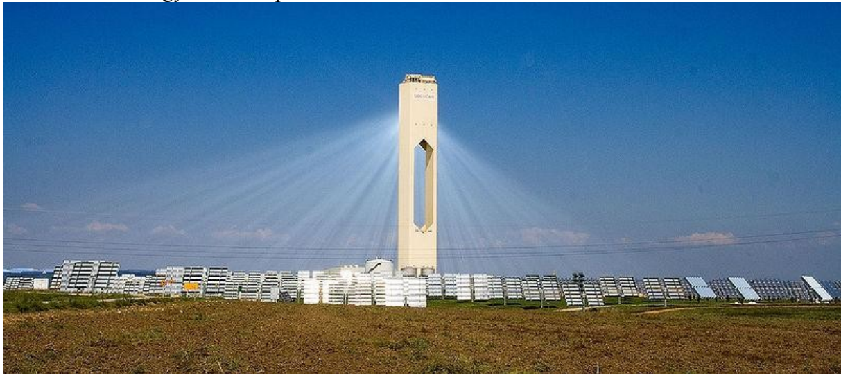
The picture shows the solar tower, where the parabolic mirrors on the ground are focused on.
