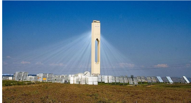
Solar tower onto which the sunlight is focused.
